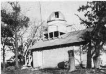
"Here is my observatory with the UNITRON 3" Equatorial inside. The roof is an 8 foot gilo roof which turns on 6 casters on an angle iron track."
